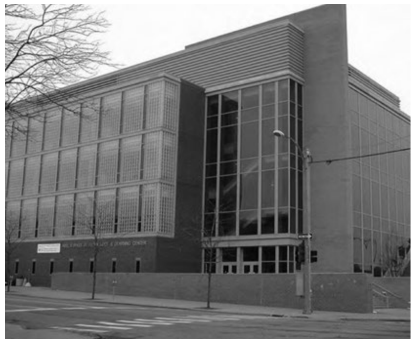
Figure 3: Applying constructability facilitates construction and reduces cost
